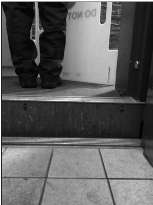
Figure 12: Elevator Car Not Levelling with the Floor
