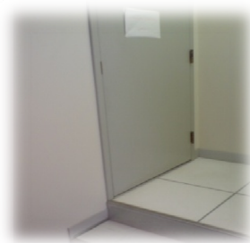
Figure 5: Exterior hinged door and raised floor
