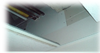
Figure 6: Access to ceiling
