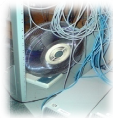
Figure 9: Fan cooling servers
