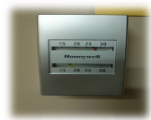
Figure 8: Temperature of server room
